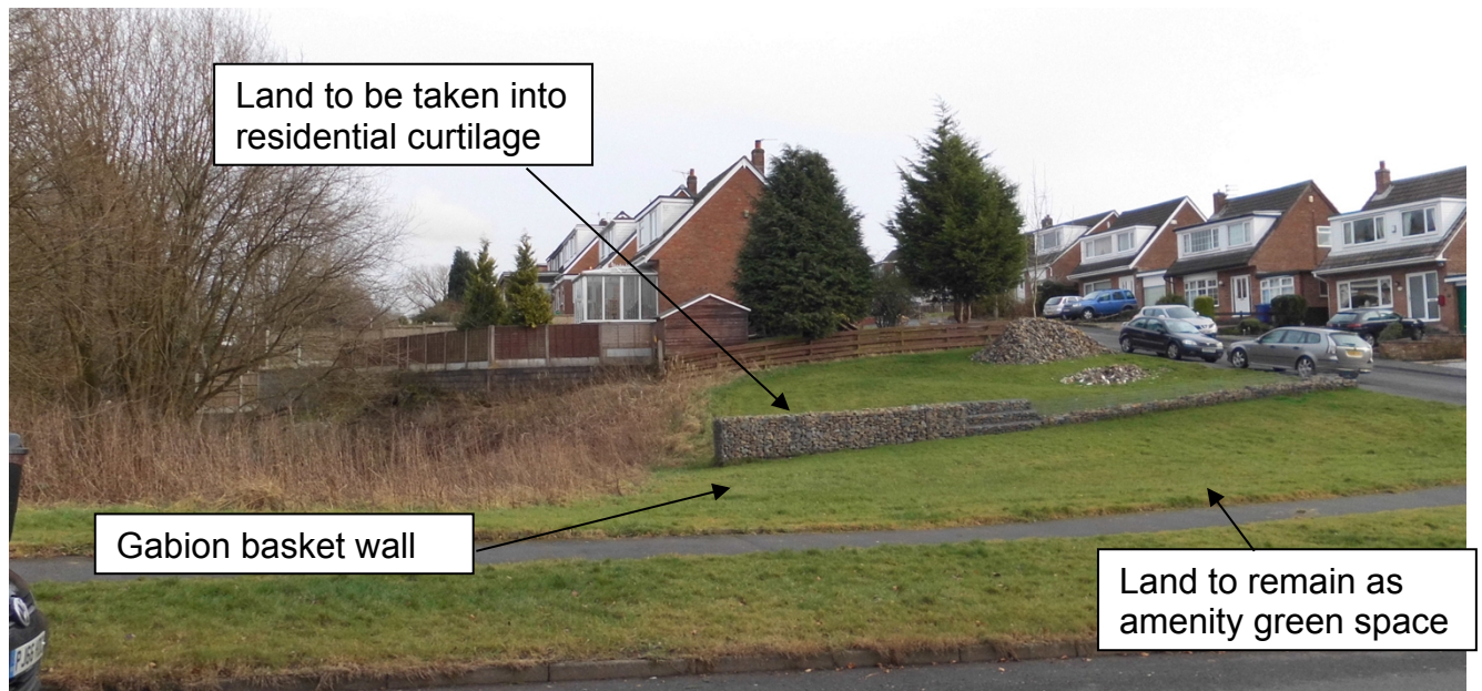
Side elevation of dwelling and adjacent land
