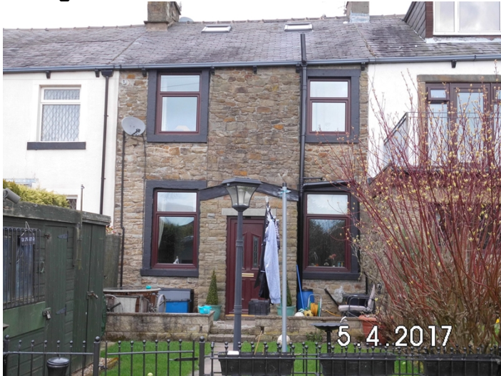
Existing frontage of application property
